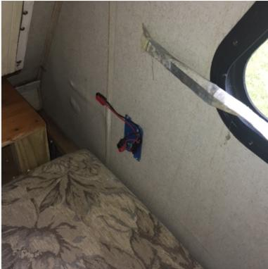
There are two 12vdc 30-Amp power pole connectors provided at the front passenger side. The total current is limited by a 30A fuse which is located near the battery in the propane/battery hood.
